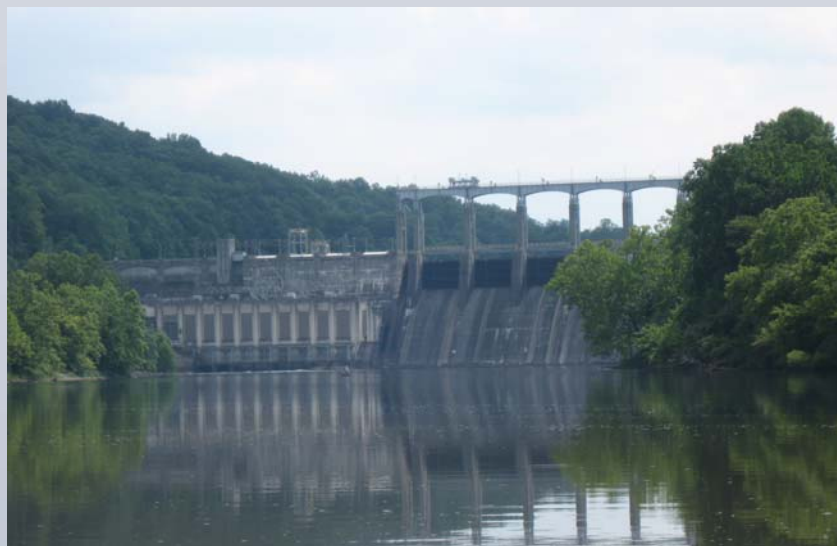
Hydro Electric Dam at Claytor Lake
